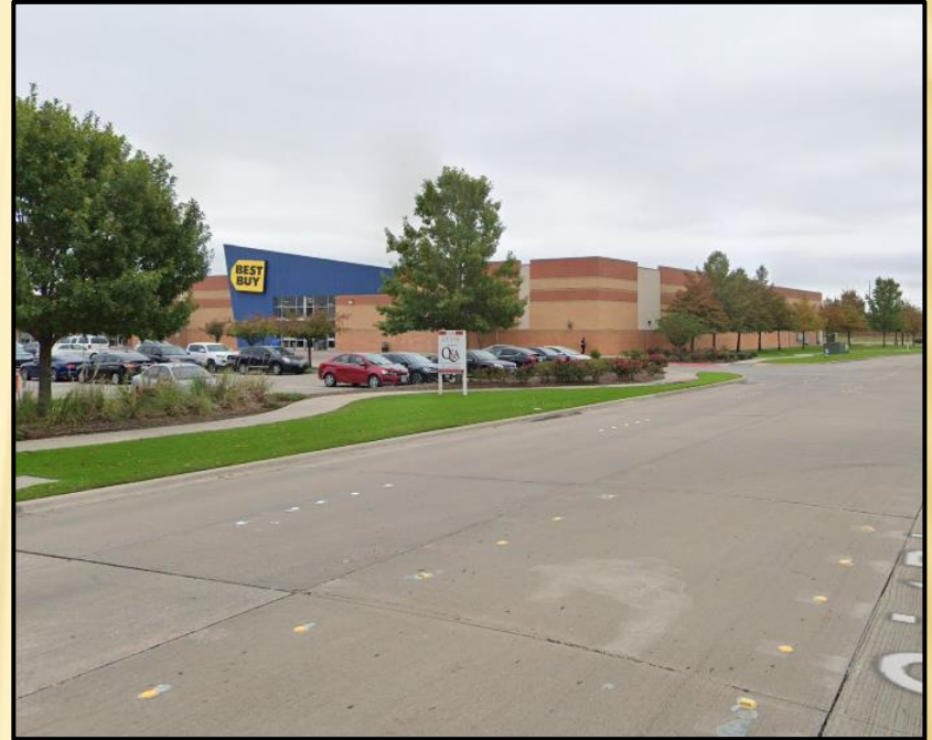
View of the property to the east.
