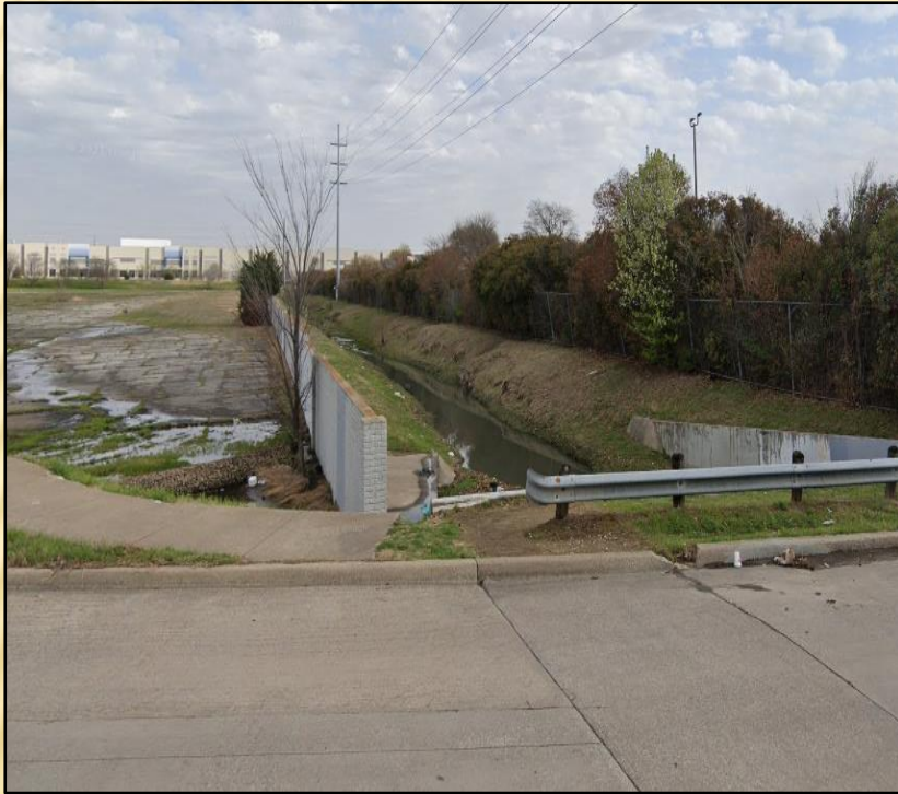
Existing Wall, drainage creek, and a dense row of vegetation.
