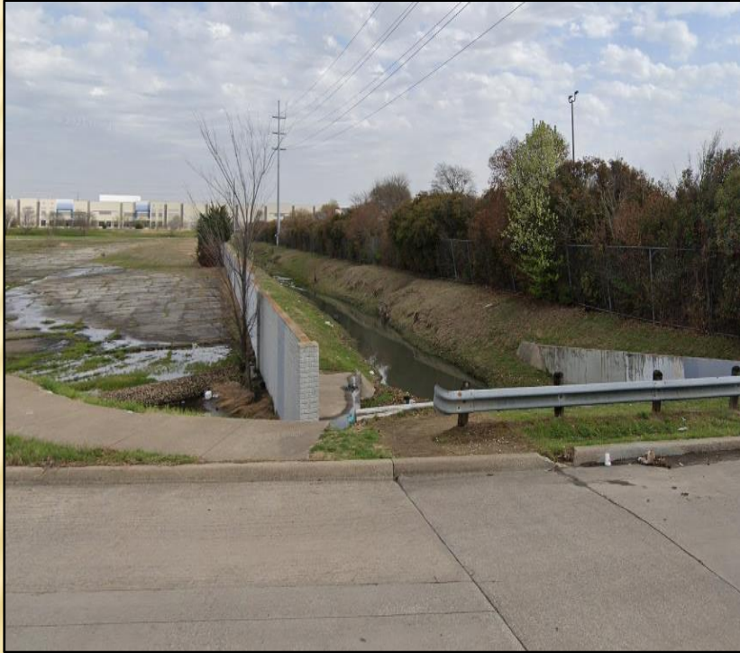
Existing Wall, drainage creek, and a dense row of vegetation.
