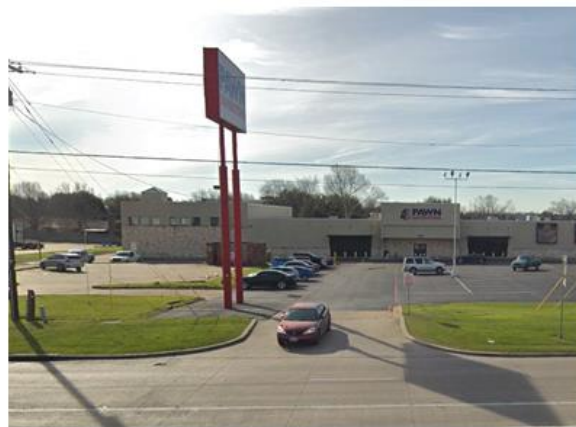
View of subject site from the north
