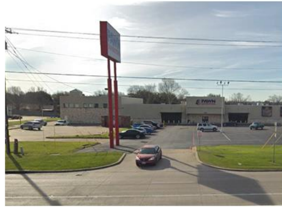
View of subject site from the north
