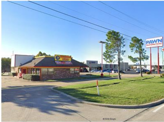
View of the adjacent property and subject site from the frontage road looking southwest
