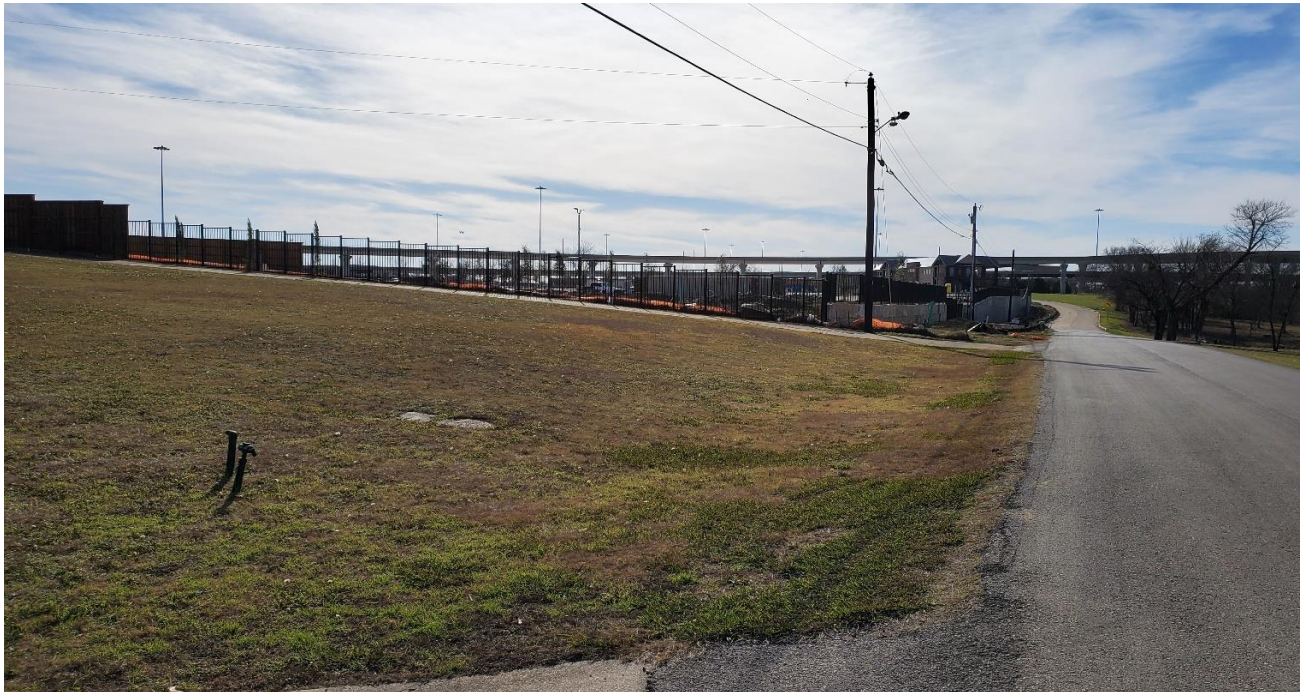
Fig 1: The current view of Phase II from Zion Road:
