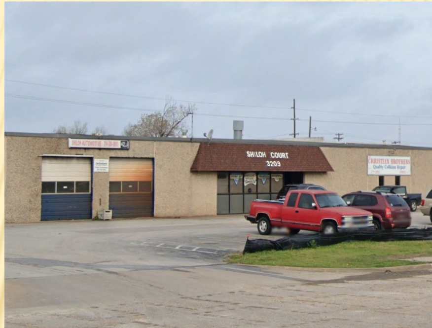
Building on the subject property along South Shiloh Road.
