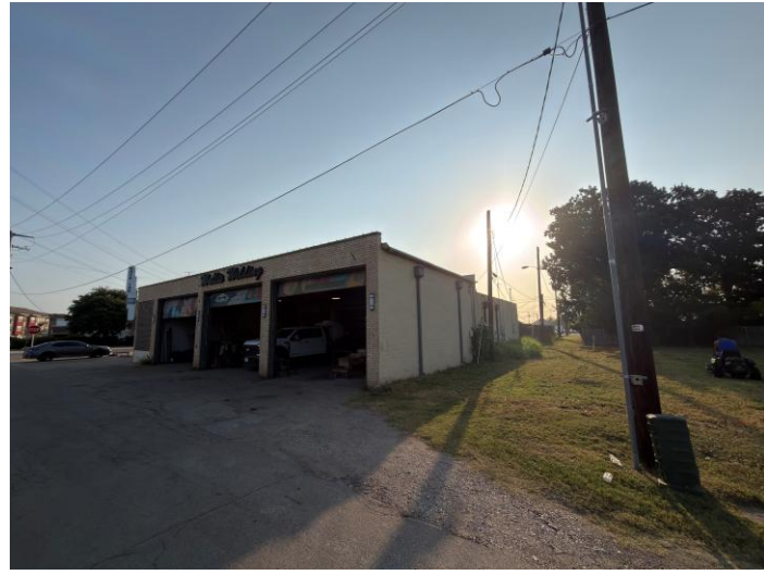
Viewing site from Southwest Corner
