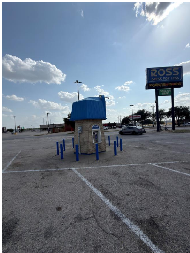
Viewing site from Southeast side
