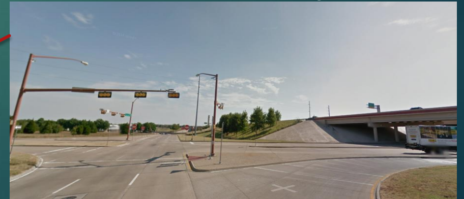
View South Along SH 190 Service Road North of Lookout Dr.
