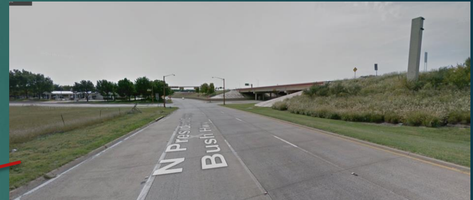
View from Middle of Site South Along Service Road
