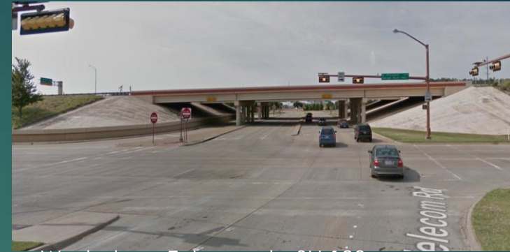
View West along Telecom to SH 190
