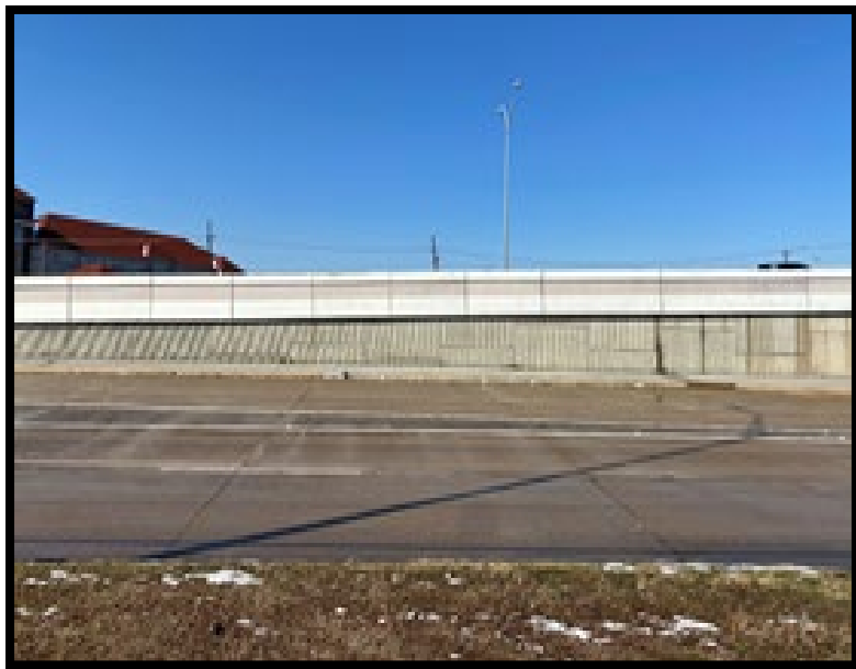
View of IH 30 and service road from subject property.
