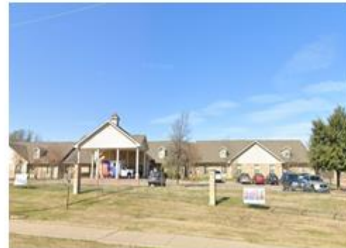
West of the subject property.
