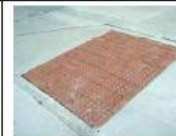
TYPICAL STREET TRUNCATED DOME PAVERS
