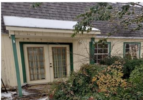
South side of the Guest House
