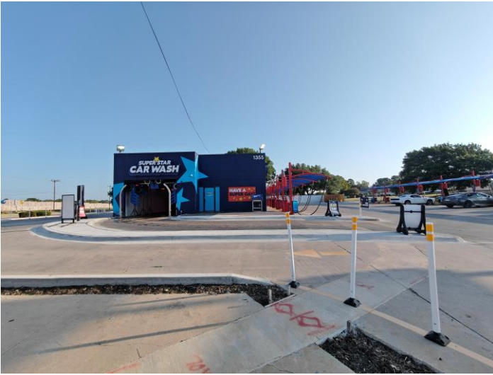
Viewing site from South side
