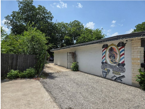
Existing dilapidated chainlink gate
