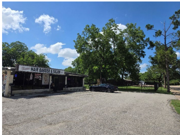
Facing North from Saturn Rd
