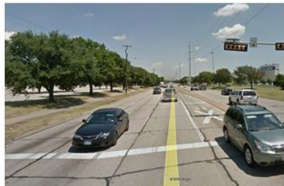
View along South Garland Avenue looking north near intersection of Leon Road Bypass
