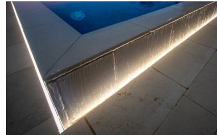
⑥ CONCEALED LINEAR LIGHTS - Outlines water feature, but is concealed from view
