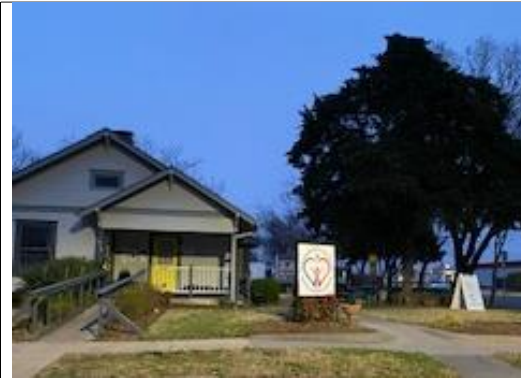
Looking at subject property from Twelfth Street
