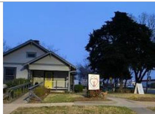
Looking at subject property from Twelfth Street
