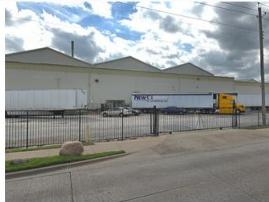
Midblock view of site on Forest Lane
