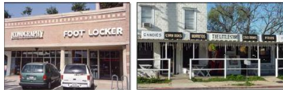
Building on the left has individually internally lit letters and are permitted. Building on the right has internally lit sign boxes which are prohibited.
