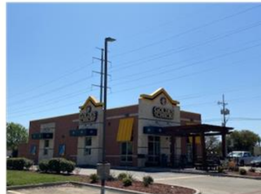
Looking south of subject site from North Jupiter Road
