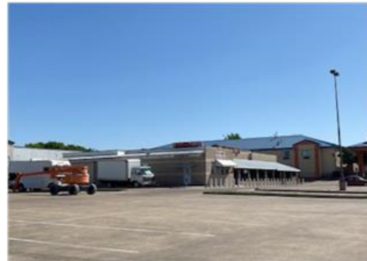
Looking east of subject site from North Jupiter Road
