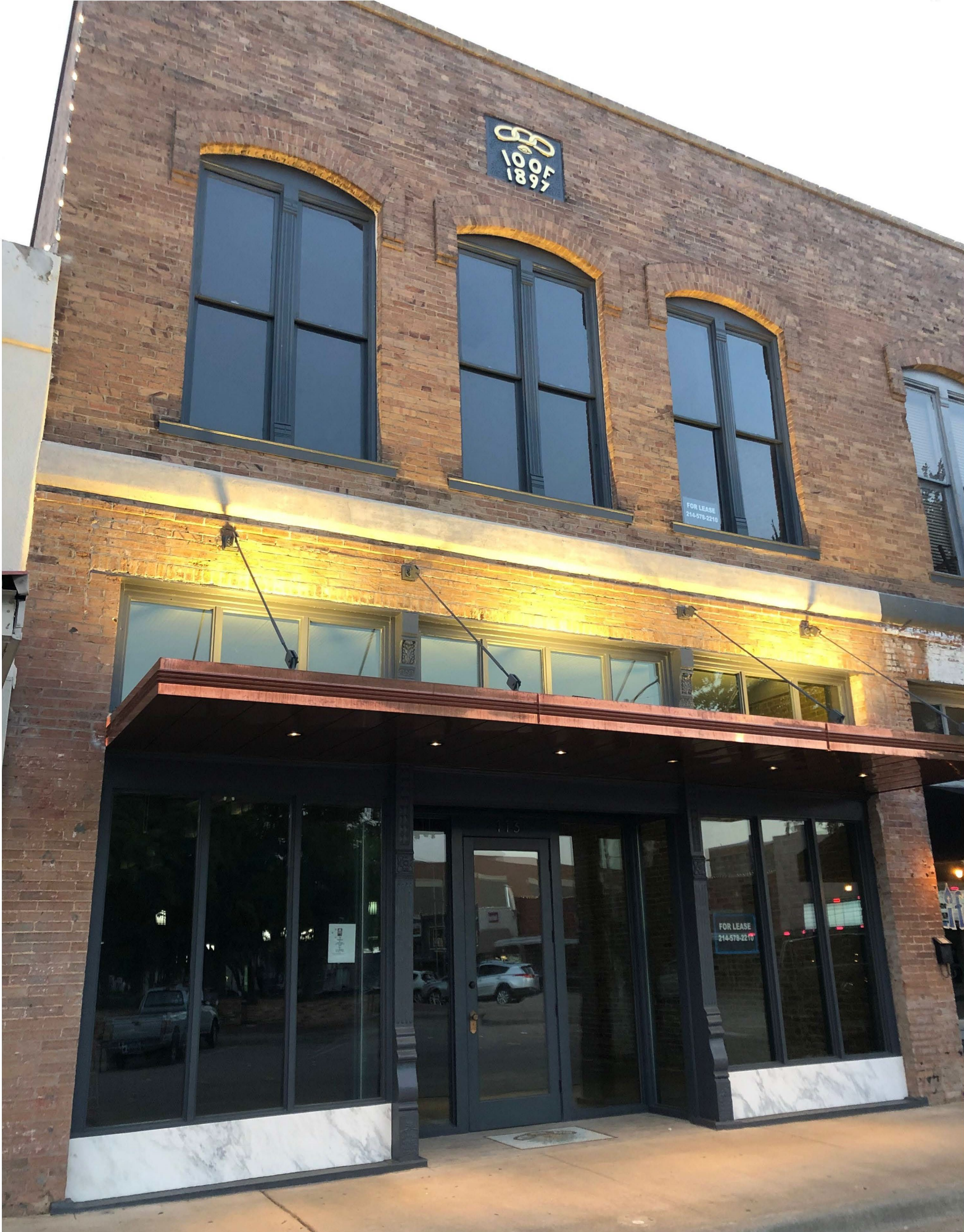
After – Renovated IOOF Building
