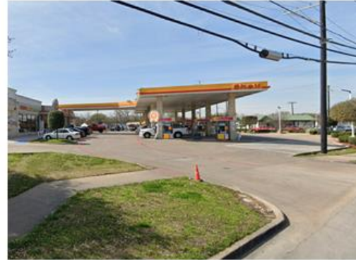
Looking west of the subject property
