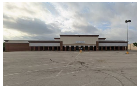
Front Building Facade
