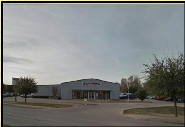
View of the subject property from Broadway Blvd.
