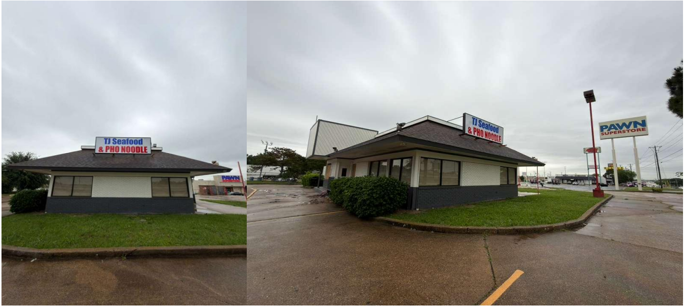
Facing South viewing site
