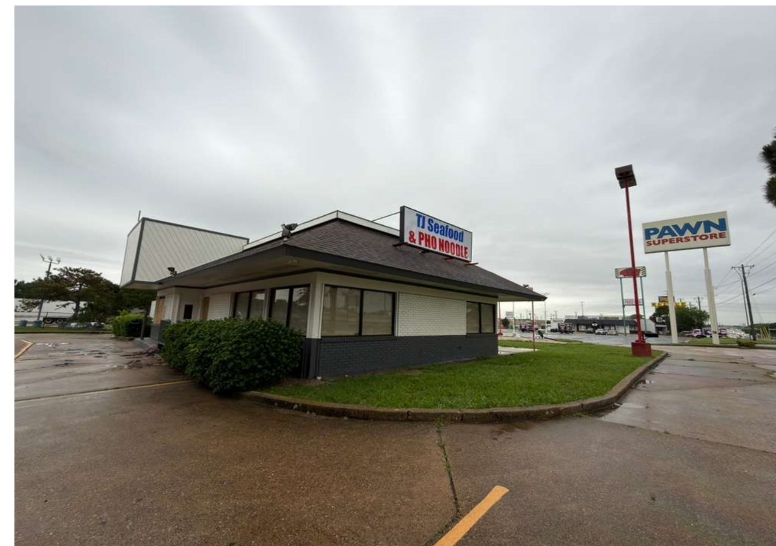
Facing South viewing site
