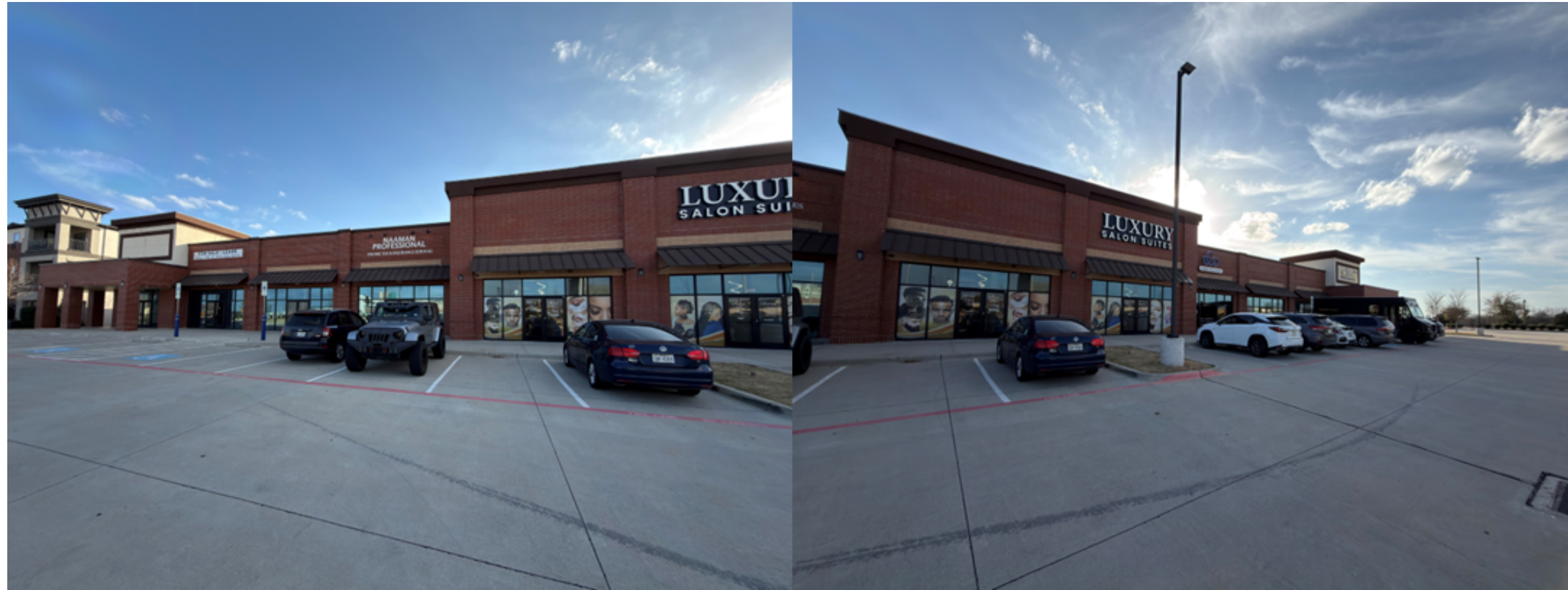
Facing South viewing site
