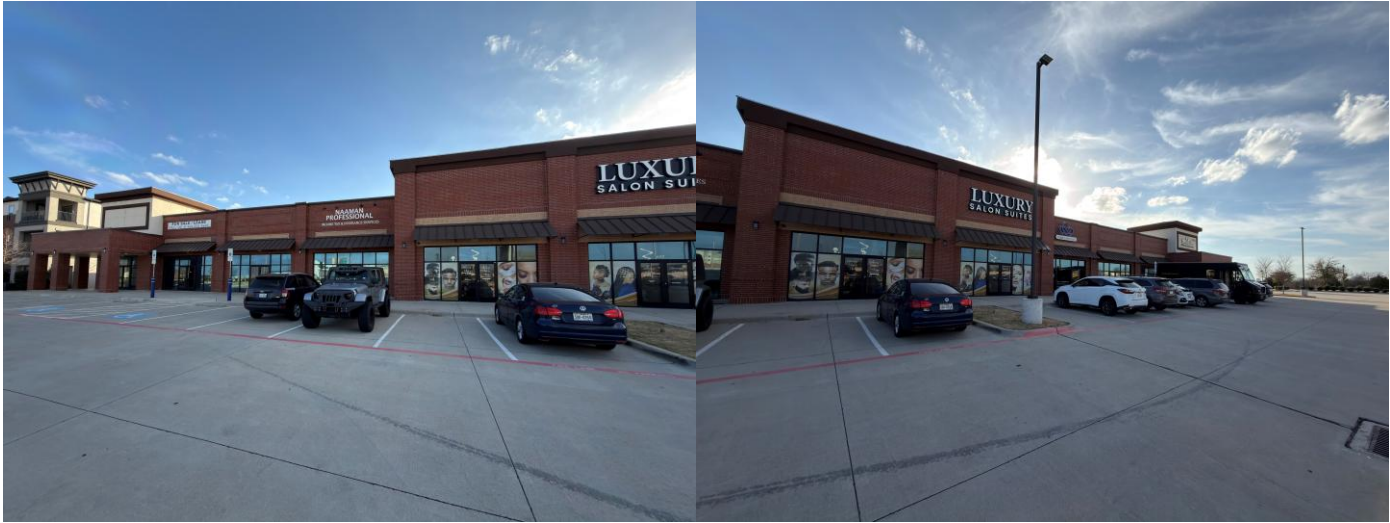
Facing South viewing site
