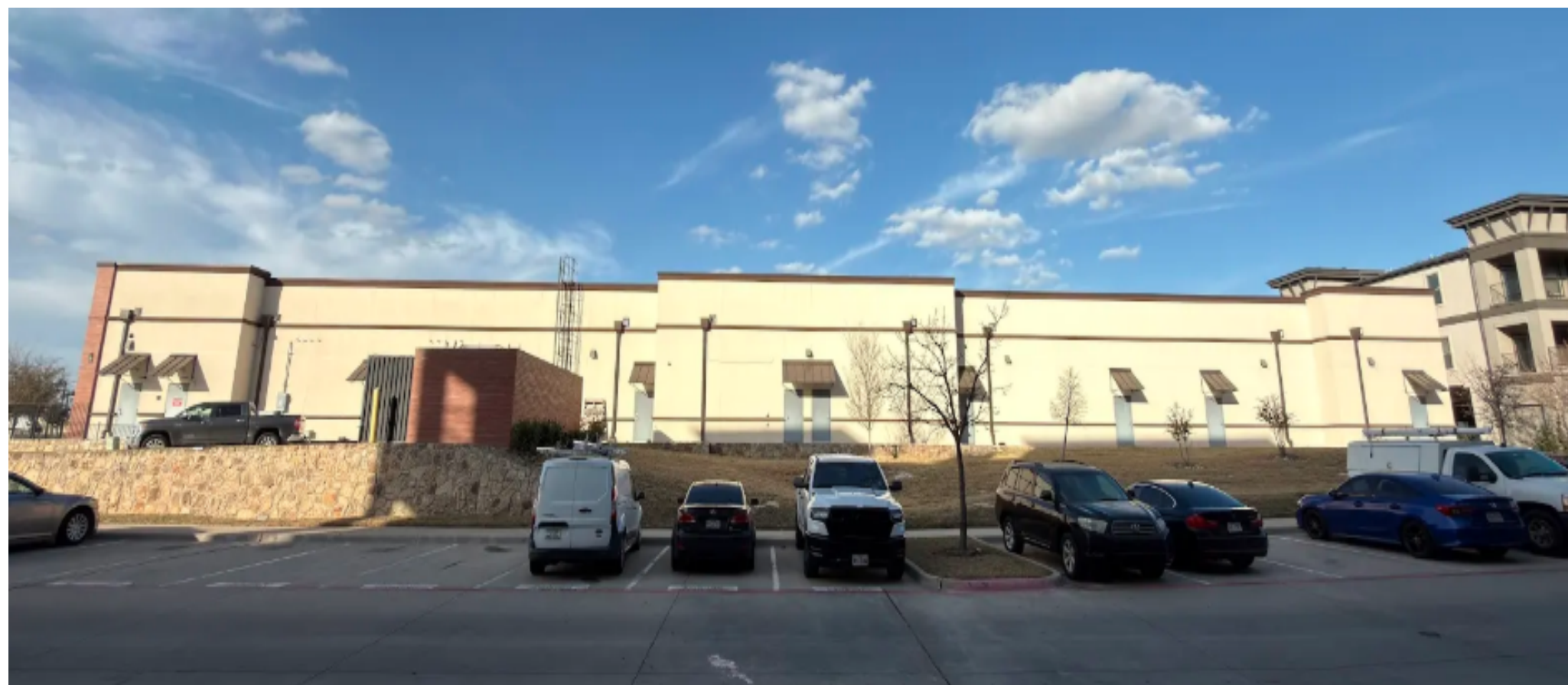
Facing North viewing site
