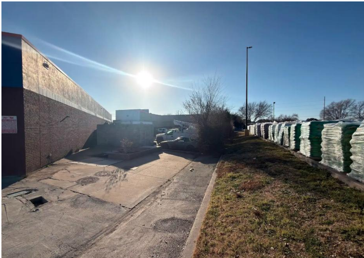
View of site facing southwest
