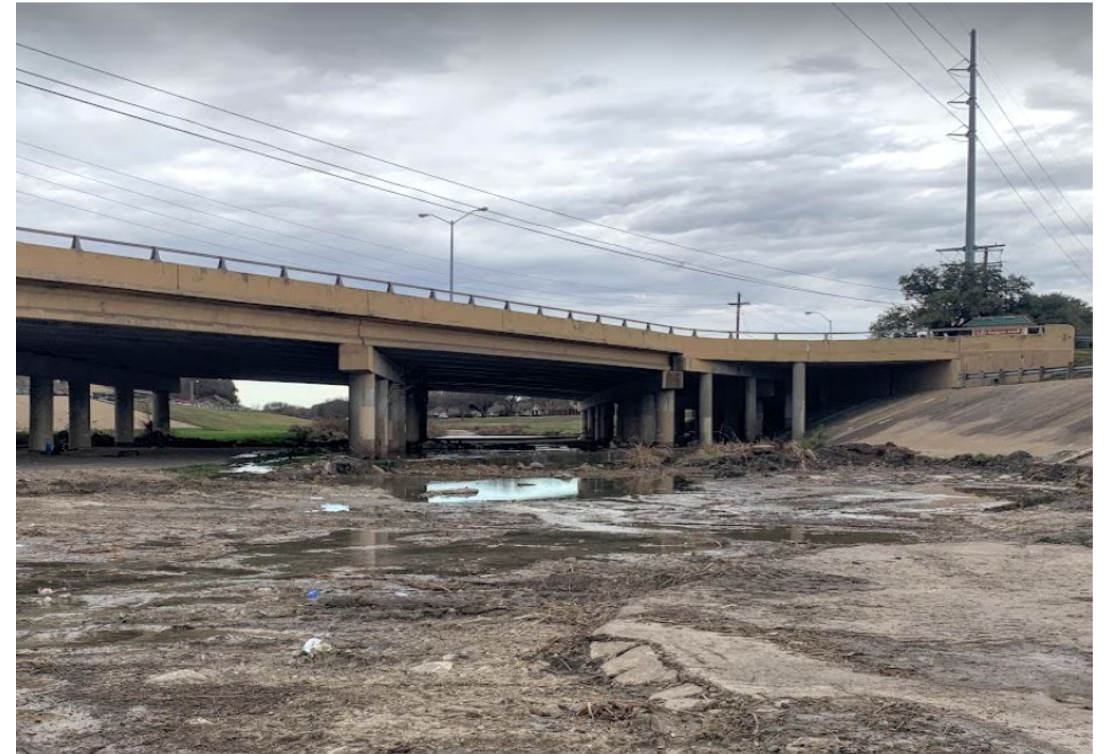
Existing conditions beneath the Jupiter Road bridge, view looking toward Richardson.
