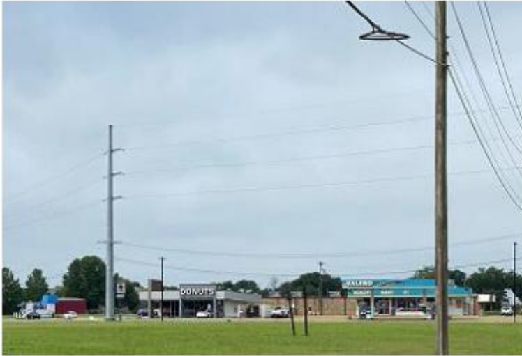
Southwest of the subject property
