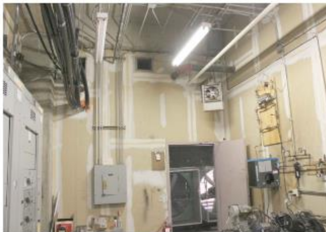
① SITE PHOTOGRAPH
