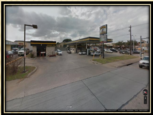
Looking at subject property from Northwest Highway
