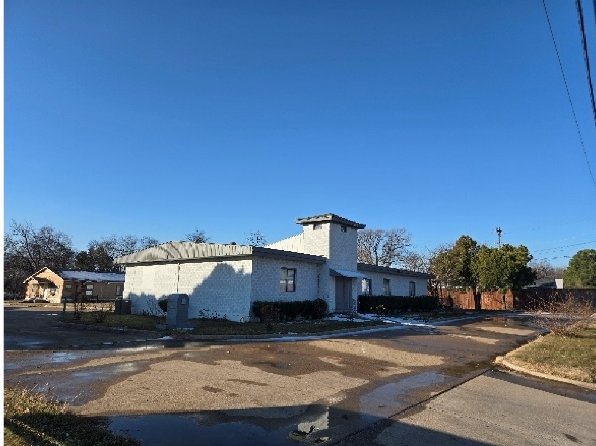
Facing south viewing back of main building
