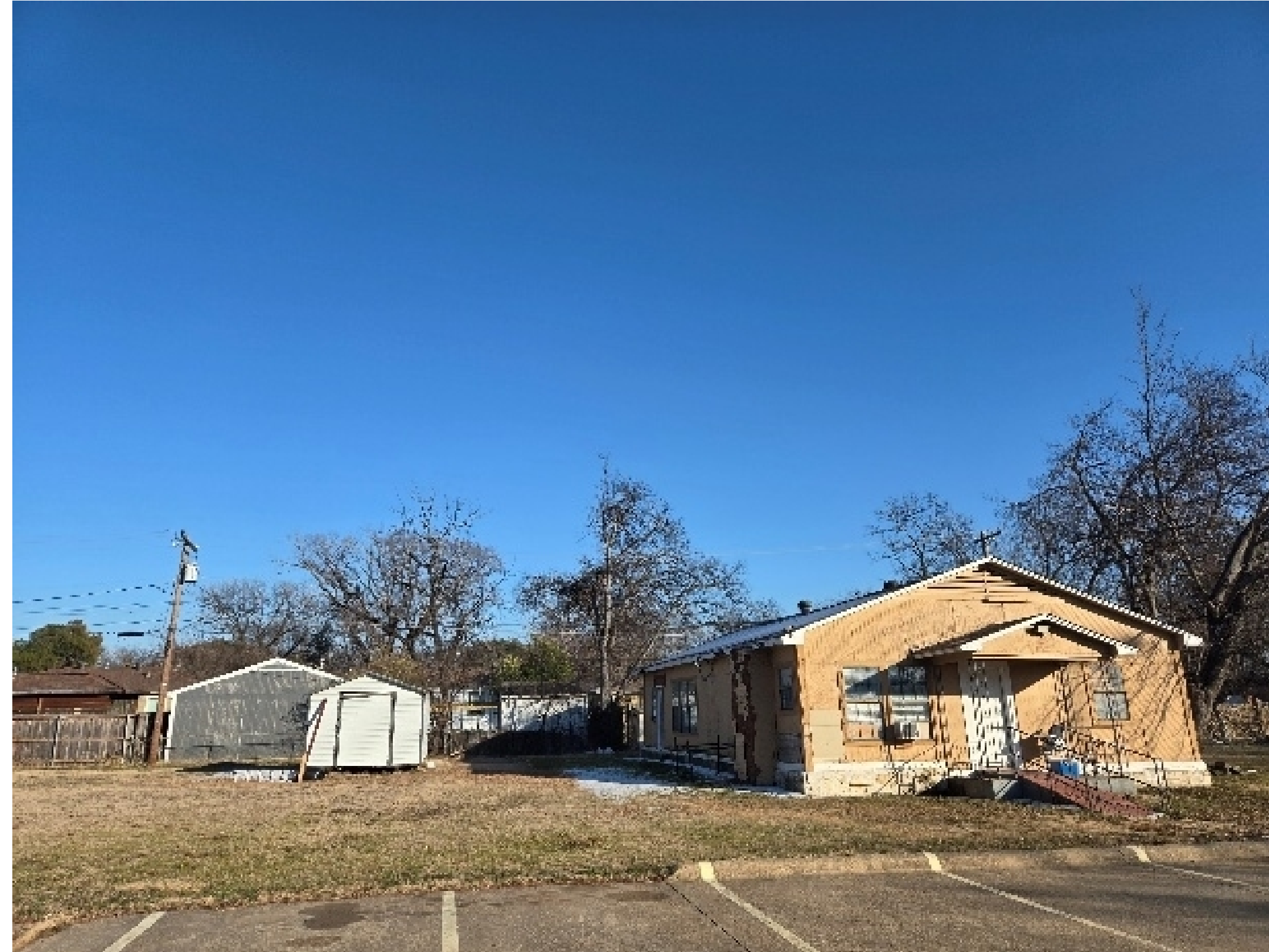
Facing east viewing the second and third buildings
