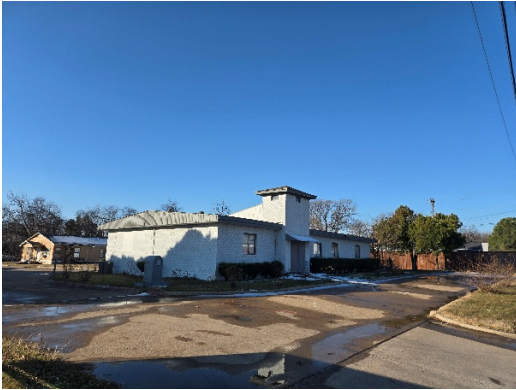
Facing South east viewing site
