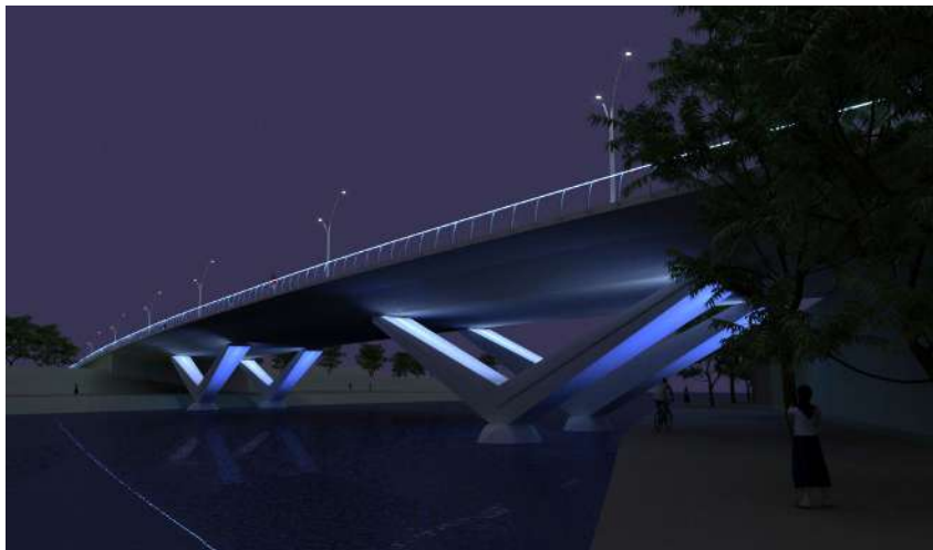
Signature Bridge (Fort Worth, TX)
