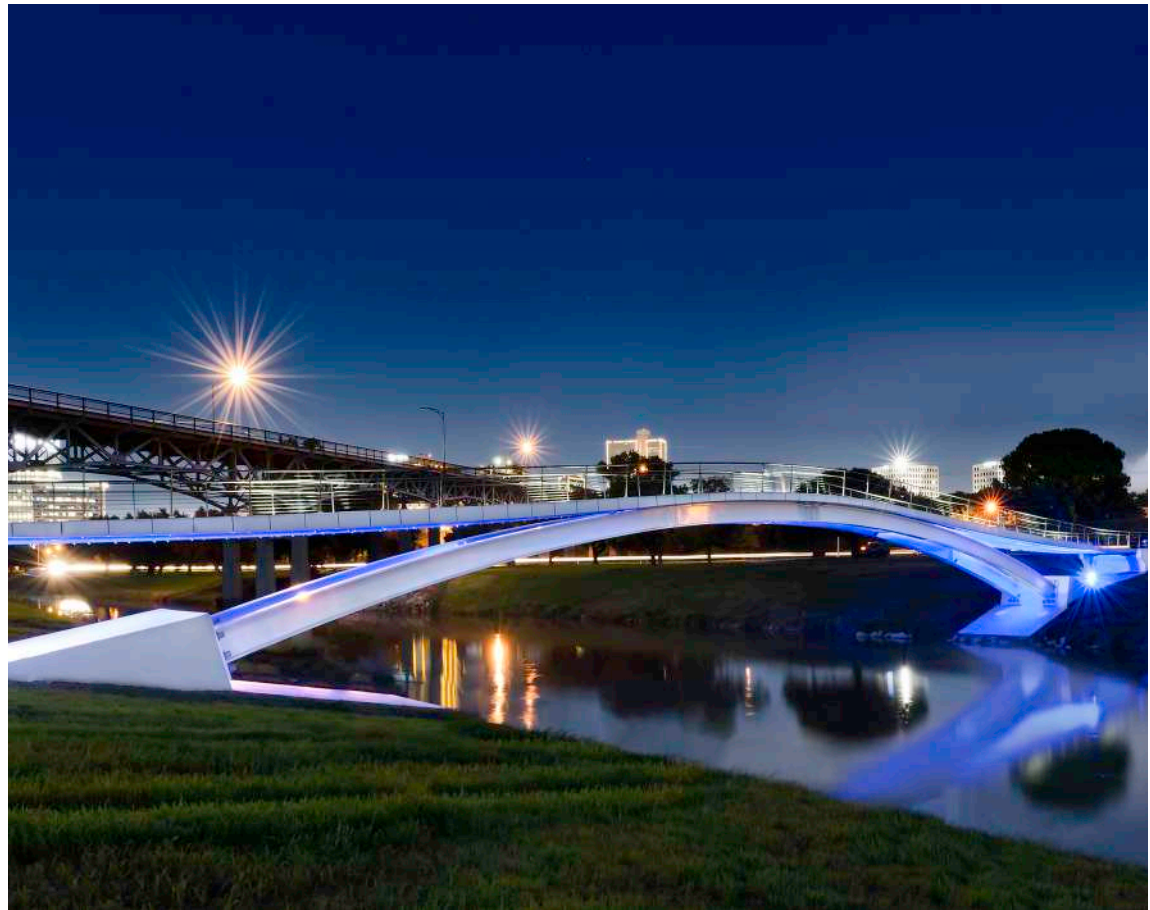
Phyllis J. Tilley Memorial Bridge (Fort Worth, TX)
