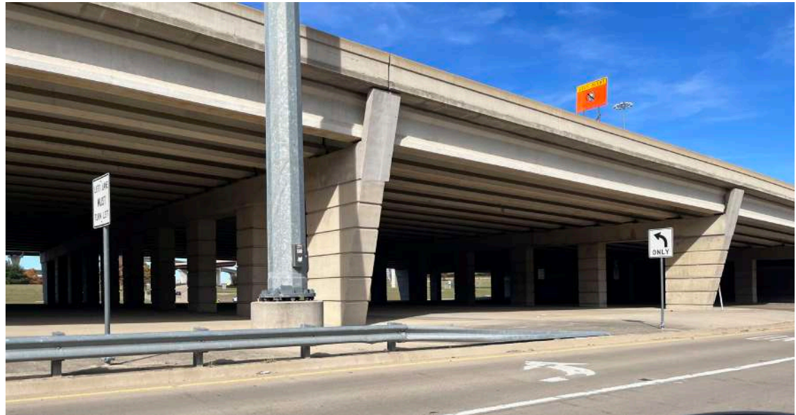
Existing I-30/PGBT Interchange
