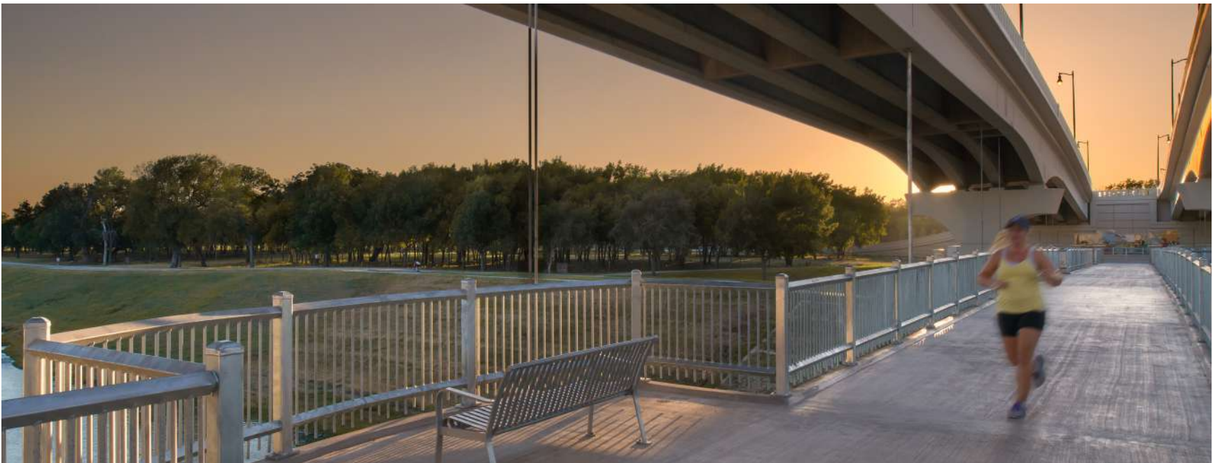
Clearfork Main Street Bridge (Fort Worth, TX)
