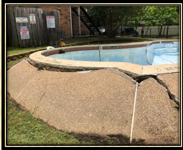
View of the existing swimming pool
