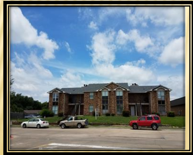
View of subject property from Apache Drive
