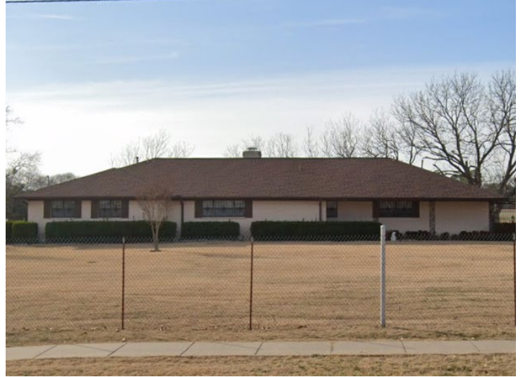
View of the southern lot with the single-family detached home.
