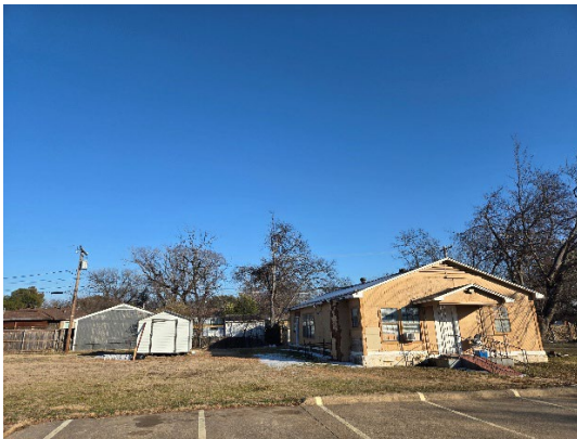
Second building and shed on site
