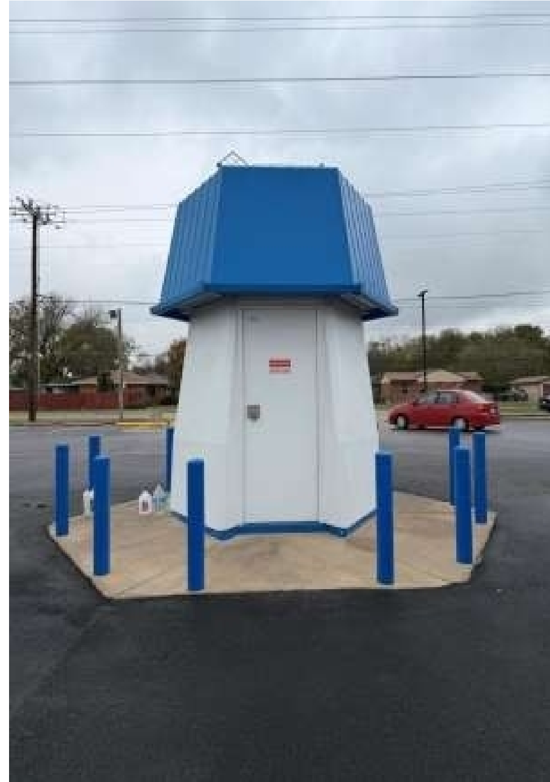
View of site facing West
