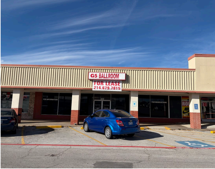
View of the suite within the shopping center.
