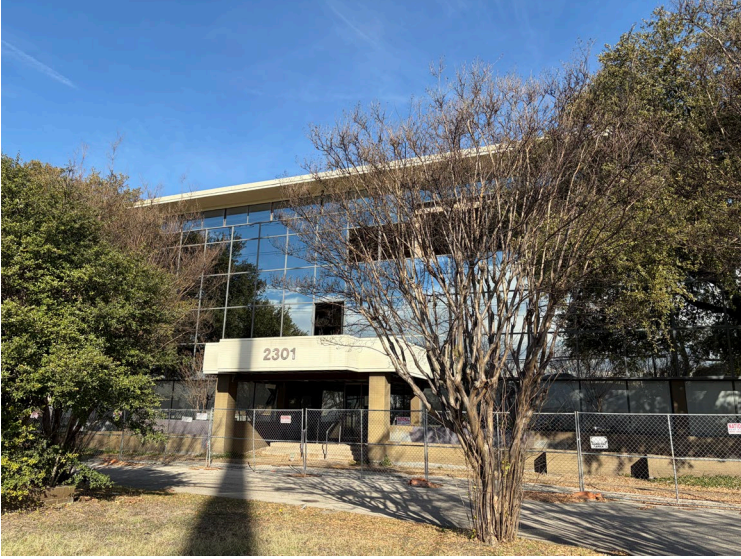
View of the existing office building from Forest Lane.
