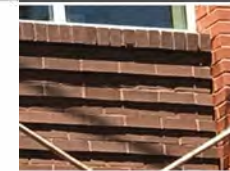
Staggered Brick Detail
