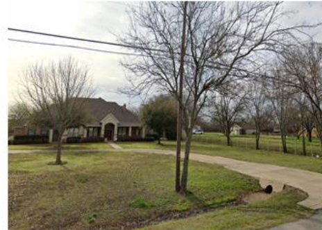
Looking west of the subject property
