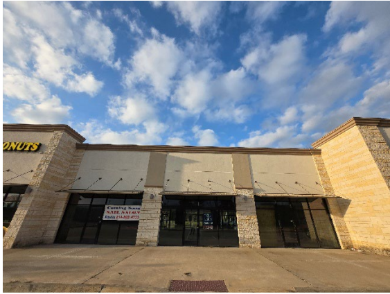
Facing North viewing site
