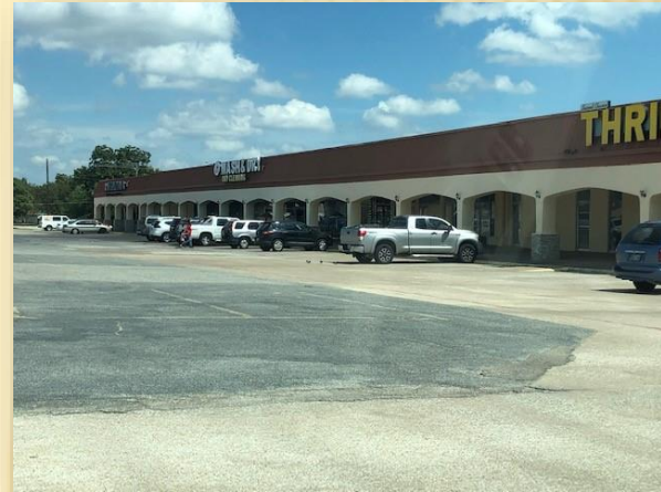
Subject commercial building
