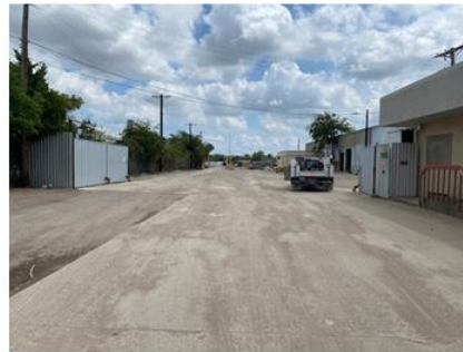
View from north entrance of the subject property
