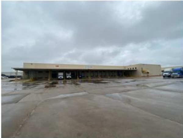
Looking at the front building, internal to the property
