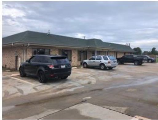
Looking at the subject property from Broadway Blvd.
