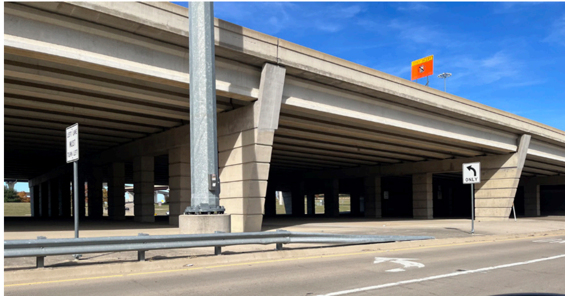
Existing I-30/PGBT Interchange
