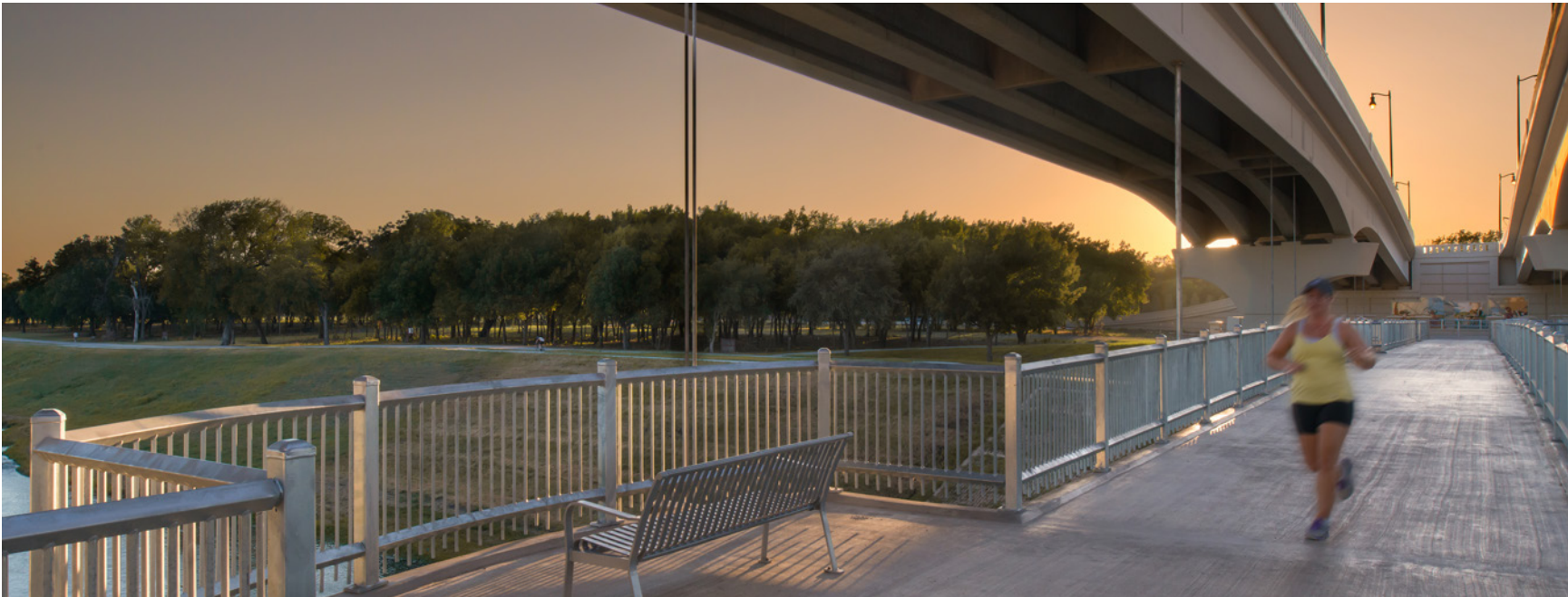
Clearfork Main Street Bridge (Fort Worth, TX)
