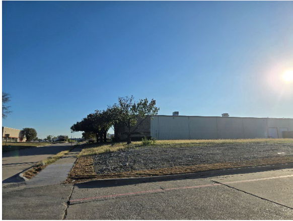
Facing South viewing site
