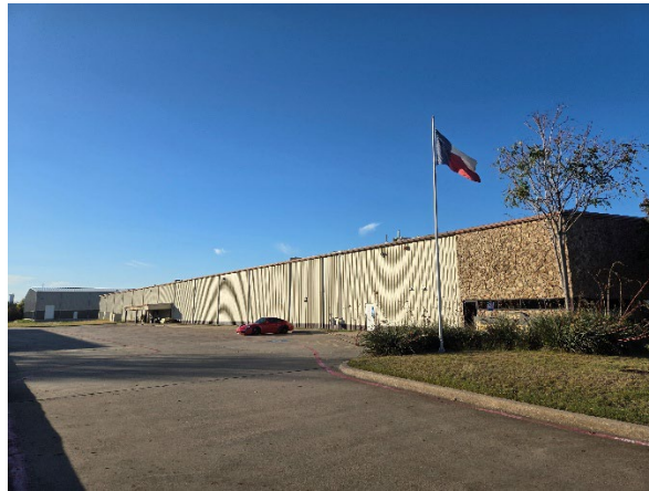
Facing North viewing site
