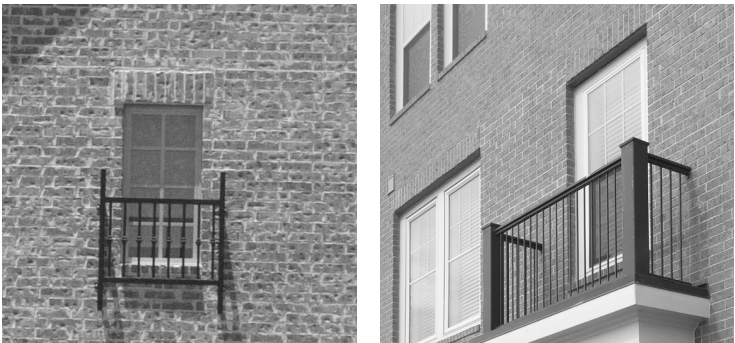
Balcony railings in front of windows are inappropriate.
