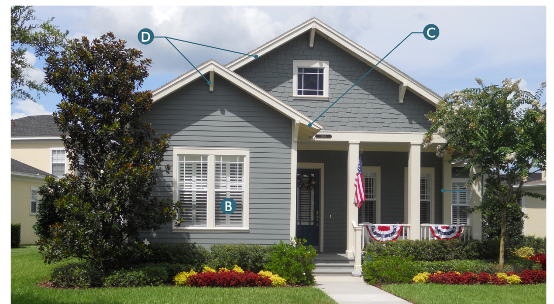
A Tapered square columns with a brick or stone base; B Ganged windows; C Deep eaves with exposed rafters or rafter tails; D Deep rake with decorative brackets; E Shed Dormer
