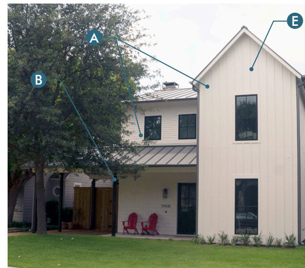
A Combination of multiple cladding materials or material applications; B Simple exposed structural members; C Shallow pitched shed roof; D Single pane fixed window; E Modern interpretation of traditional form
