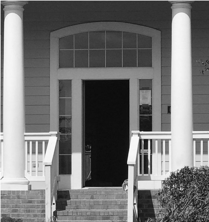
Over scaled transom is too tall in proportion to the primary entrance door.
