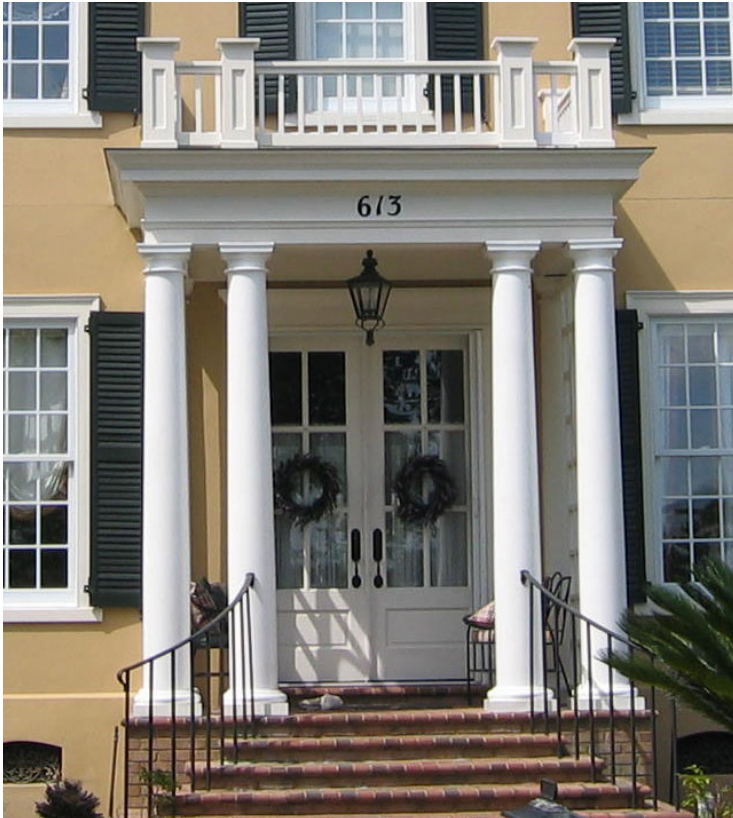
Over scaled transom is too tall in proportion to the primary entrance door.
