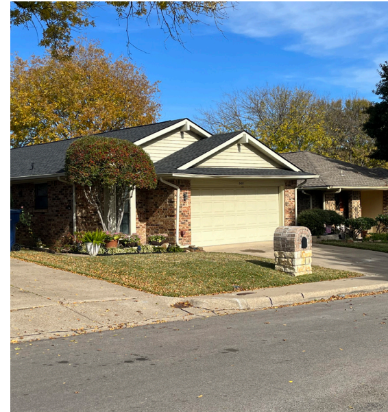
Existing Windsurf Bay Residential
