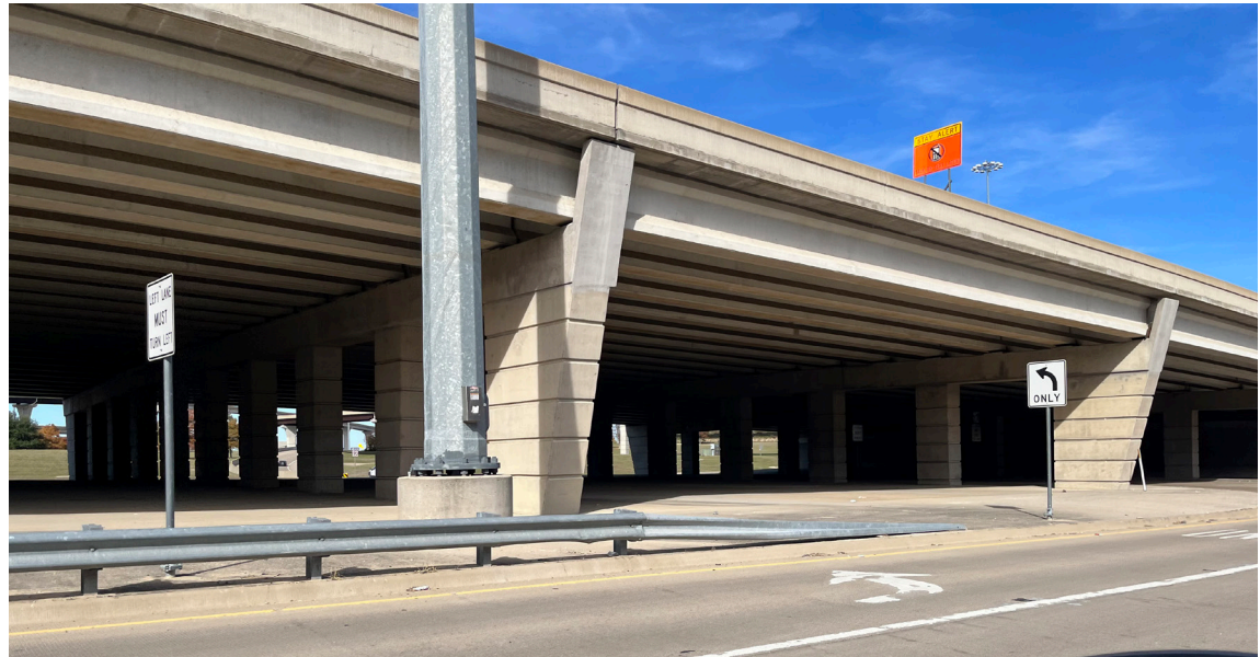
Existing I-30/PGBT Interchange
