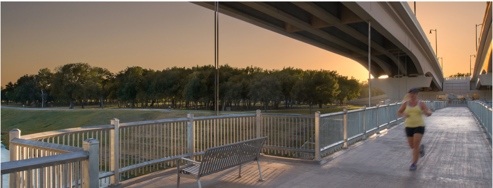
Clearfork Main Street Bridge (Fort Worth, TX)
