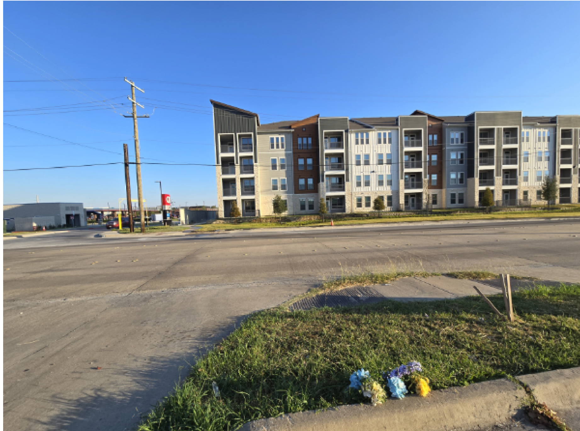
View from subject site facing north
