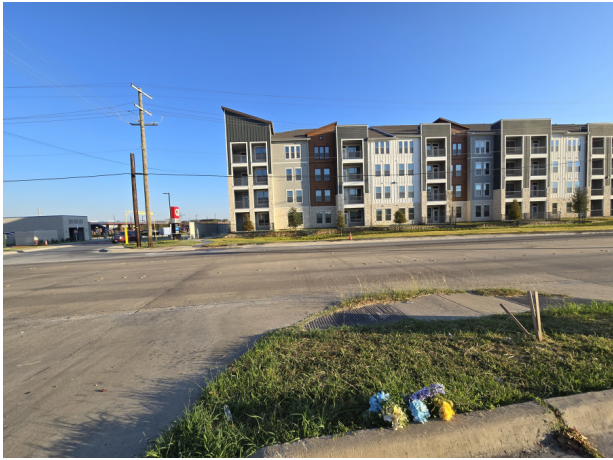
View from subject site facing north
