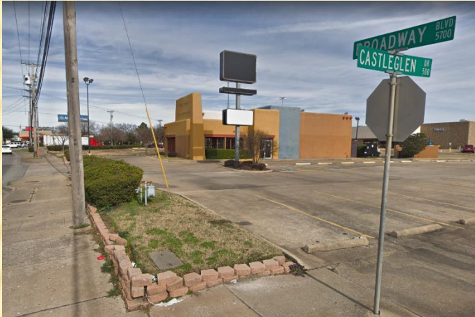
View from the corner of Castleglen Dr. and Broadway Blvd. of existing structure.
