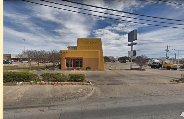
View from Broadway looking north towards the existing structure.
