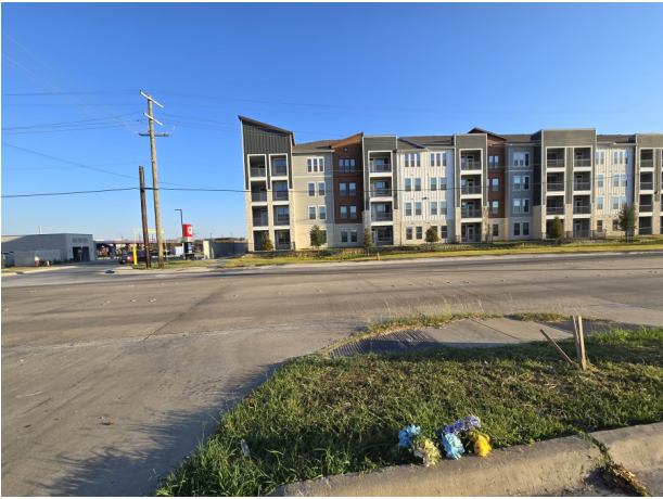
View from subject site facing north
