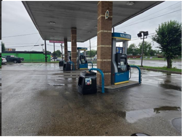
Photo of fuel pumps facing south
