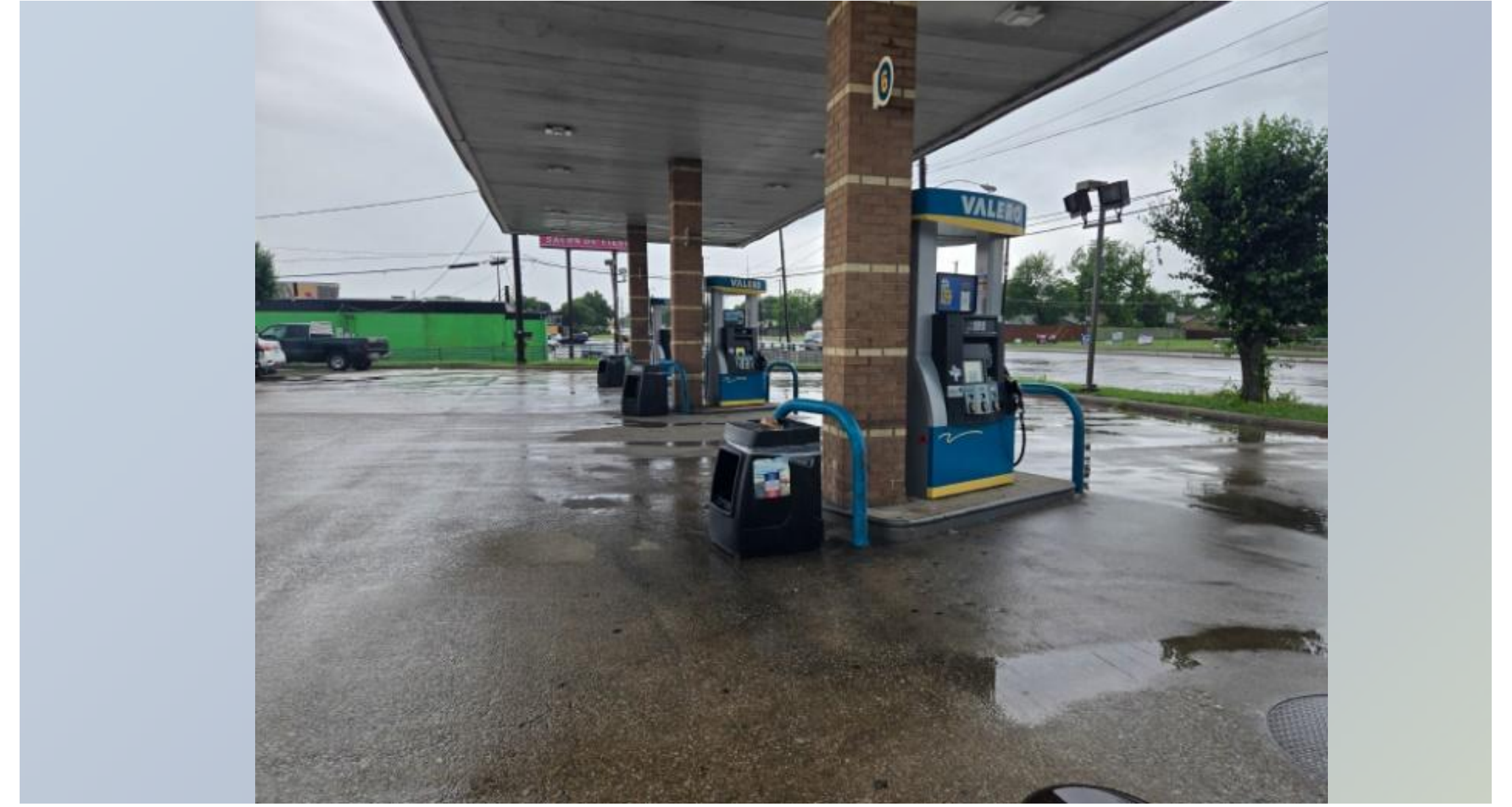
Photo of fuel pumps facing south
