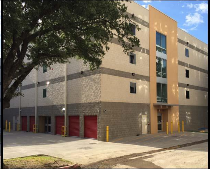
No access gate
