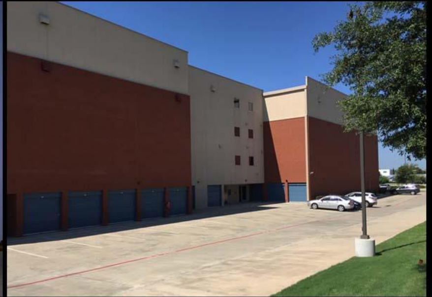
No access gate
