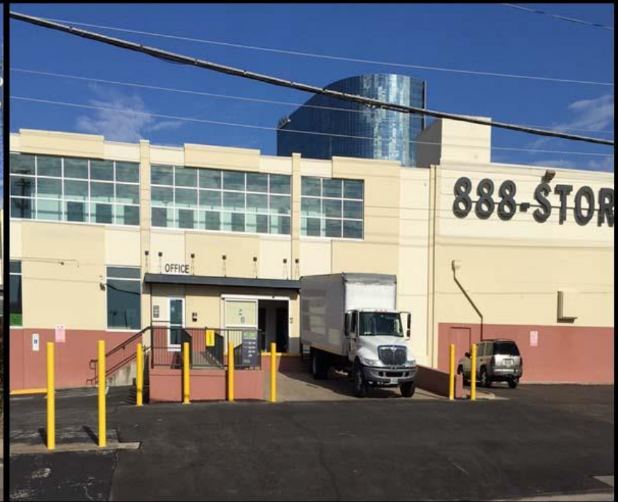
No access gate
