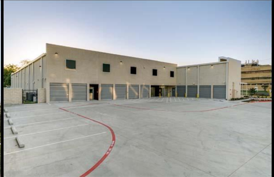
No access gate
