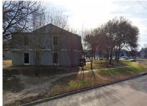
Looking west of the subject property
