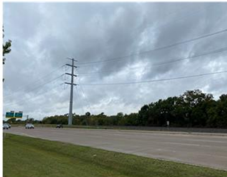
Looking west of the subject property from Lavon Drive
