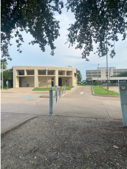
View from the southeast along Edgewood Dr
